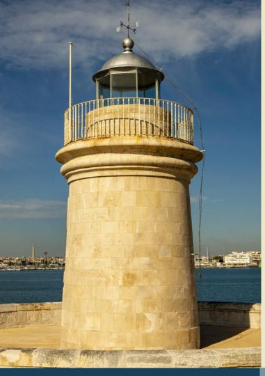
This ancient and small lighthouse was built in 1879, on the northern end of the breakwater, after the sinking of a sailing vessel which in the storm failed to overcome the pier, ending up against the rocks. It was built right on the ancient Bourbon pier of which it represents the only remnant.
